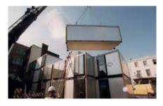
Three dimensional units produced in a factory that are transported to site and bolted together. The frames will normally be steel, timber or concrete and can be supplied with all external and internal finishes (including services such as electric and plumbing)
